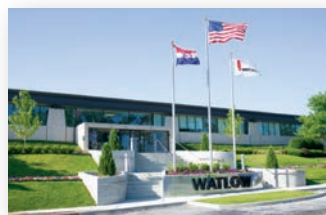
1995 Watlow headquarters following two expansions
