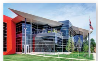
2016 Watlow's headquarters and Advanced Technology Center following a complete renovation
